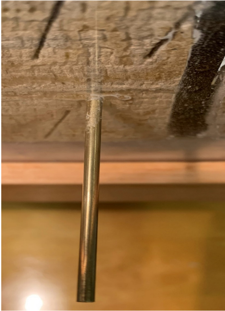
Figure 3, brass bearing rod underneath the subroadbed
